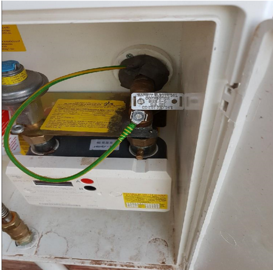
Holding bracket shear bolts ground off after meter has been fitted.
