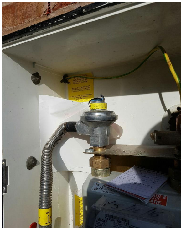
Foam put in spigot Hole wrong material used this should be Plumbers mastic putty. Do not use Pink fire retardant foam as a sealant.
