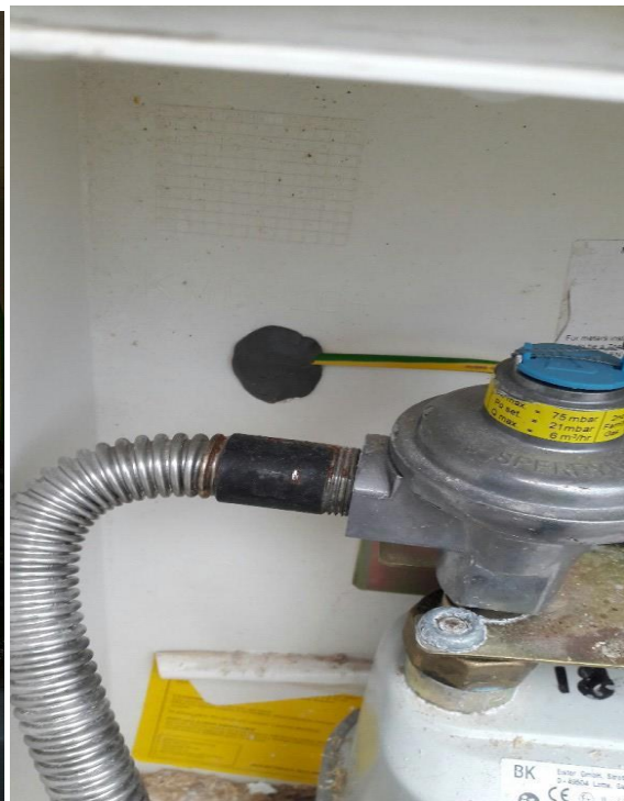
Foam put in spigot Hole wrong material used this should be Plumbers mastic putty. Do not use Pink fire retardant foam as a sealant.
