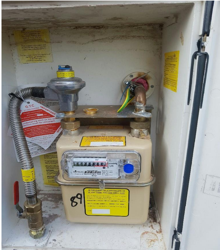
Foam put in spigot Hole wrong material used this should be Plumbers mastic putty. Do not use Pink fire retardant foam as a sealant.
