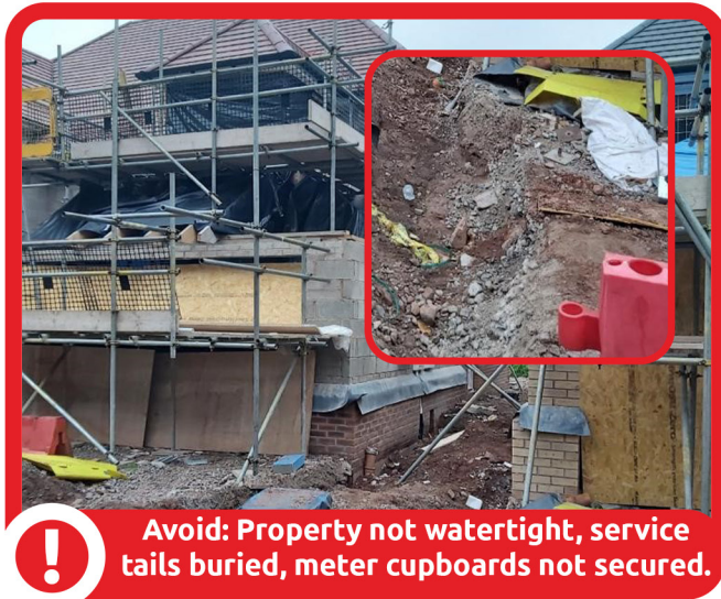
! Avoid: Leaving meter cupboard un-installed - cannot connect.
