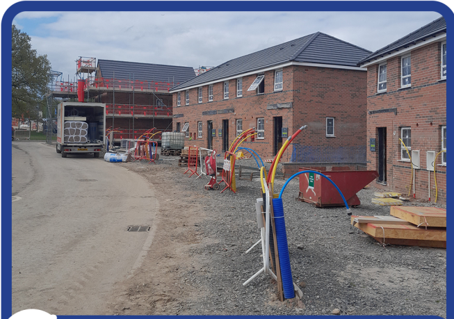
✓ Access unobstructed, water-tight, boxes installed & secured, tails showing.
